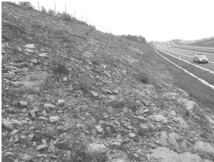
Fig. 2: The slope planting with the cuttings of succulents and grass-herbal seeds
