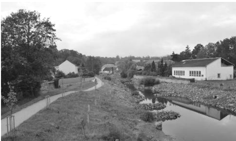
Fig. 1: View of the modified riverbed of the Blanice River in Vlašim - newly built stone shoots in the riverbed, shore fortifications, planting of woody vegetation and landscaped walking trail (Lampartová, 2016)
