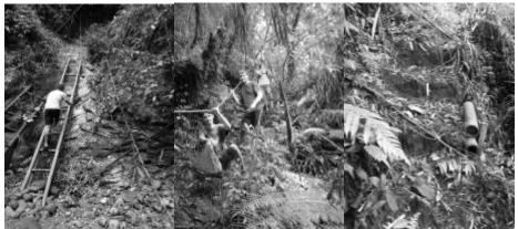
Fig. 5: Stabilization of the trails: Bamboo ladder (bottom of the river valley), Using secure top-rope construction, Lengthwise lateral bamboo stabilizations of path stairs
