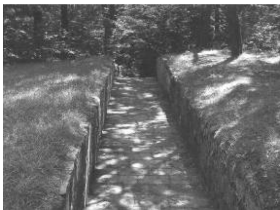
Fig. 3: Safety stone weir of the water reservoir Počúvadlo (Source: author's archive)
