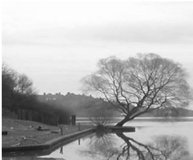
Fig. 1: Passive stabilization, Brno reservoir, „OSADA“ area, foto M.Šlezinger, 2011
