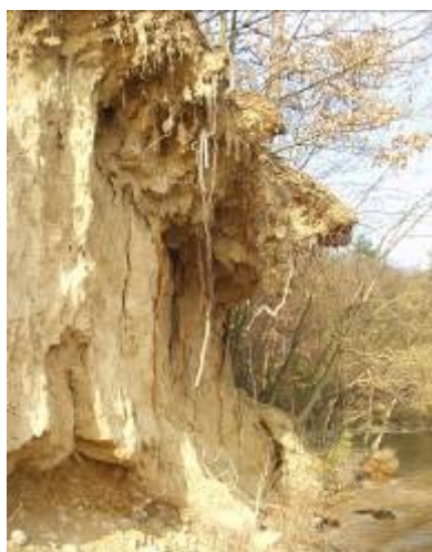
Fig. 2 Overhanging platform over an erosion wall - Brno reservoir, „OSADA“ area, foto M.Šležingr, 2011
